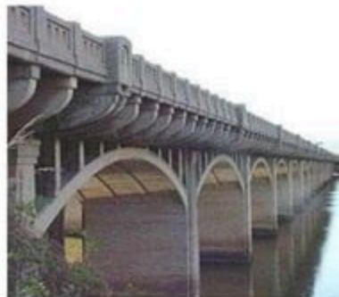
Monolithic Concrete Arch
