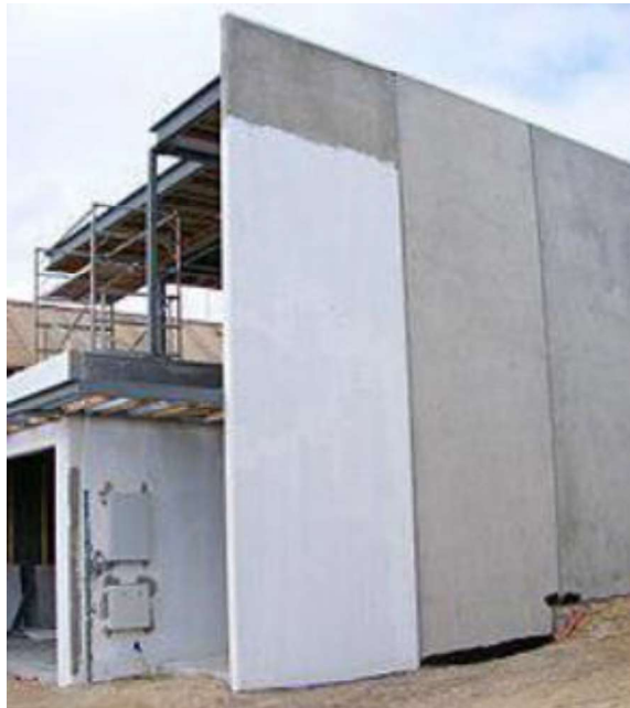
A house being built with prefabricated concrete panels.
